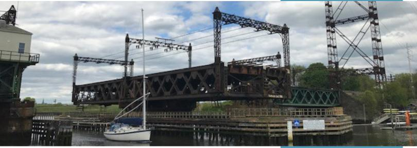
The existing Walk Bridge (Bridge No. 04288R, MP 41.5), constructed in 1896, carries four railroad tracks and approximately 175 trains and 125,000 passengers daily. One of the oldest movable bridges on the Northeast Corridor, the 564-foot long, four span swing bridge has outlived its lifespan. The Walk Bridge has been subject to continued operational failures and vulnerable to damage from harsh weather conditions and requires replacement.
